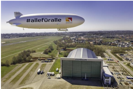
Zeppelin Hangar © Michael-Haefner
